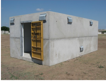
Above Ground Community Shelter
